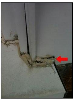
Condition: • <u>Vines</u> Implication(s): Chance of water damage to contents, finishes and/or structure | Material deterioration Location: Exterior Wall Task: Remove Time: Immediate
