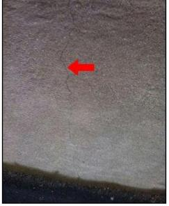
Condition: • <u>Spalling, crumbling or broken material</u> Implication(s): Weakened structure | Chance of structural movement Location: Exterior Wall Task: Repair Time: Immediate
