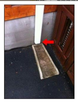
Condition: • Downspouts discharging onto roofs Implication(s): Chance of water damage to contents, finishes and/or structure Location: Exterior Porch Task: Correct Time: Immediate
