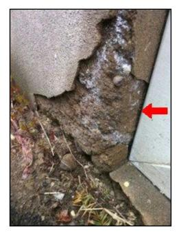
FLOORS \ Columns or piers Condition: • Poorly secured at top or bottom Should be replaced with steel post. Implication(s): Weakened structure | Chance of structural movement Location: Basement Task: Replace Time: Less than 1 year
