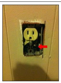
Condition: • <u>No GFI (Ground Fault Interrupter)</u> Implication(s): Electric shock Location: Exterior Wall Deck Task: Replace Time: Immediate
