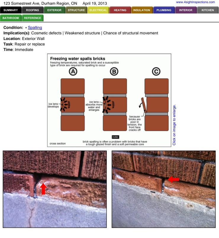
Condition: • Mortar deterioration Implication(s): Chance of water entering house | Weakened structure | Chance of structural movement Location: Exterior Wall Task: Repair Time: Immediate
