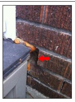
Condition: • Bolts protruding from wall Location: Exterior Wall Task: Improve Time: Immediate
