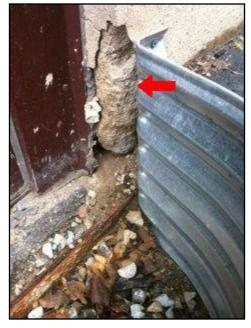
**Condition:** • Parging damaged or missing Implication(s): Chance of damage to structure | Shortened life expectancy of material Location: Exterior Wall Task: Repair or replace Time: Immediate
